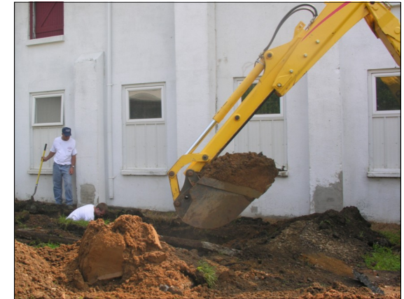
Excavating the trench
