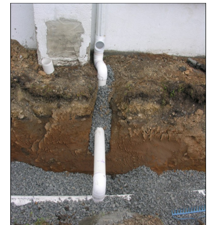
Pipes attached to downspouts and laid in trench; filling trench with gravel
