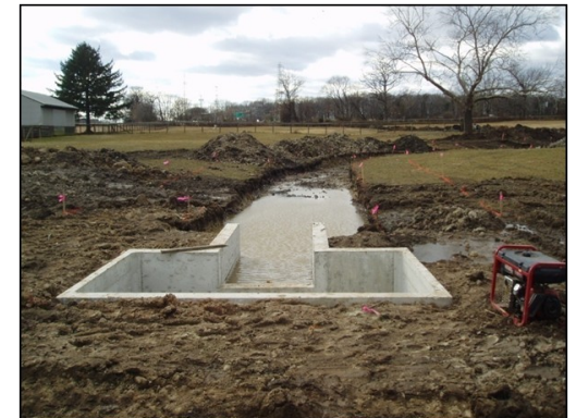
Digging the channel
