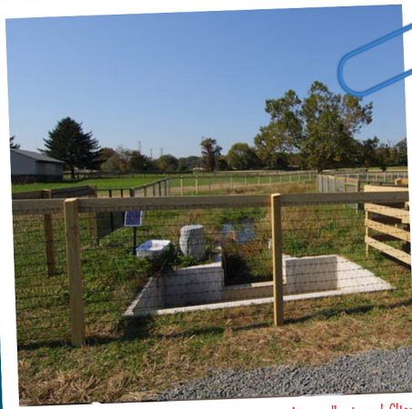
A bioswale at the Ryders Lane Farm is used to collect and filter runoff as it passes through native grasses.
