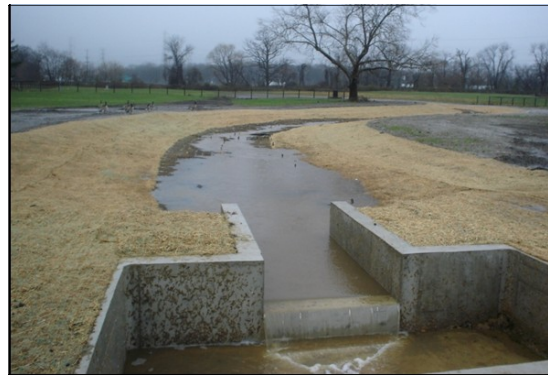
Shortly after bioswale construction
