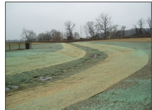
The channel has been graded, seeded, and had erosion control matting added
